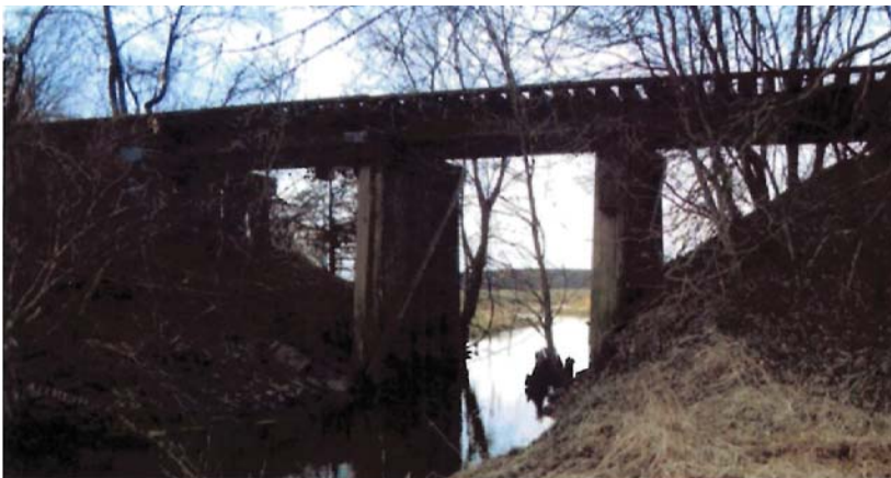
County Ditch 32 Crossing
