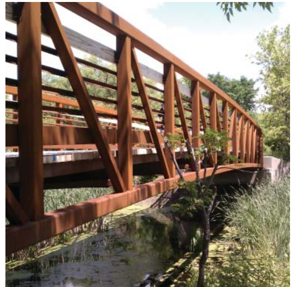
Prefabricated truss bridge for trail use.
